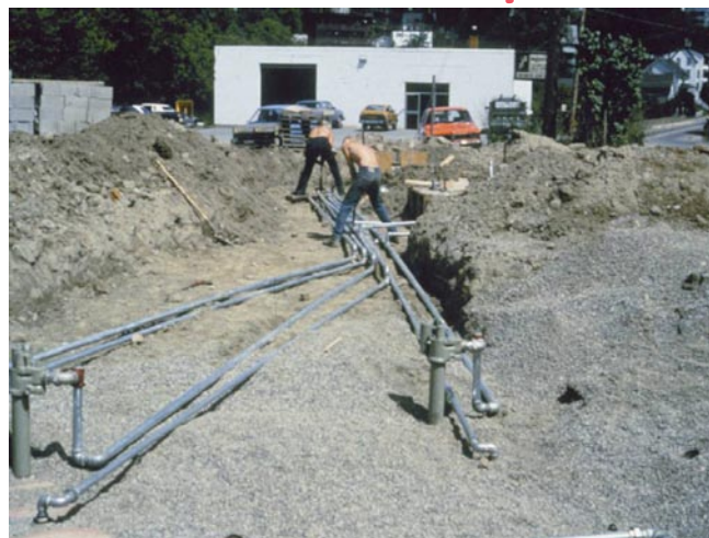
Galvanized-pipe installation from days of yore.
